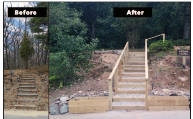
A before and after photo of the project site
